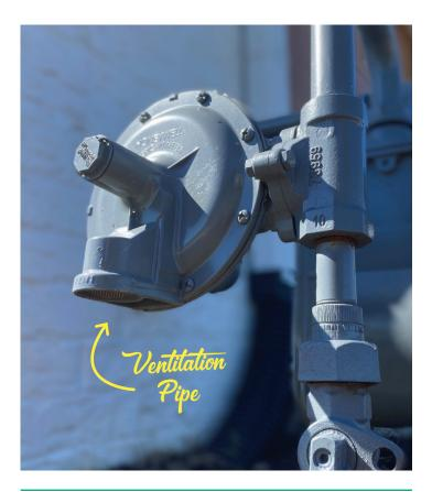
Be sure to **gently remove** all snow and ice buildup from the meter and ventilation pipes. The ventilation pipe is located underneath the saucer shaped portion of the meter equipment.
